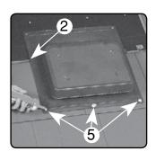
Apply sealant to the underside of the flashing ③. Install so that the next full shingle will lap over the flashing. Apply sealant at the bottom of the shingle where it meets the top of the pipe/vent ④. Apply sealant over exposed fasteners ⑤.
