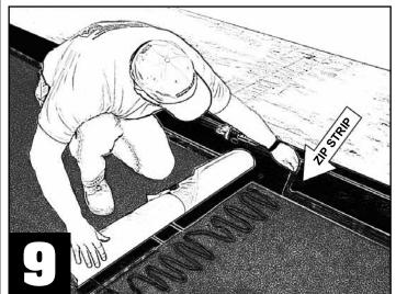
After removing the release liner be sure to remove zip strips from bottom sheet and from selvedge edge on previous course as you applying the end lap. Roll end lap to ensure a solid contact. As you continue up the roof, applying additional courses, all side laps must be 4" and end laps must be 6". To avoid lining up end laps on subsequent courses, TAMKO requires a minimum stagger of 18".
