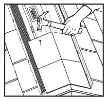
2. Place first piece of vent with female end 1" in from gable end and use centering line for proper alignment along peak. Fasten using at least two nails at each end and in the middle of section in nail line area (2-1/2" minimum nail length). More may be required on steeper slopes to seat properly. Continue installing additional pieces along ridge
