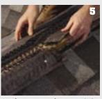
To splice, remove nylon matrix (3") as shown in photo #3 and fit together by overlapping remaining fabric with next section and fasten to roof deck.
