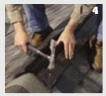
Create end cap by folding fabric in toward center at each side; then up and over nylon matrix so that it covers the end of the vent. Center Roll Vent over slot and fasten with nail lines up. Nail on nailing line.
