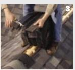
Loosen about 6" of nylon matrix from fabric and cut out with snips.
