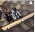
Snap chalk line and cut a slot  $3^1/2^n$  wide  $(1^3/4^n)$  on each side of ridge beam). Allow for a closed area of sheathing (with no slot) approximately  $18^n$  at both ends of ridge.
