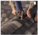
Install ridge cap shingles with even spacing on both sides of Roll Vent using 2½" in from cap shingle edge on nailing line. Nails should penetrate the sheathing a minimum of ½". Ridge cap must overhang Roll Vent by a 1" minimum at each gable end.
