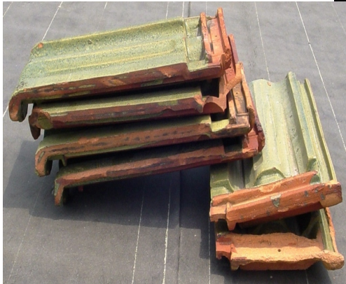
Side View - Staged Tiles (Slope →)
